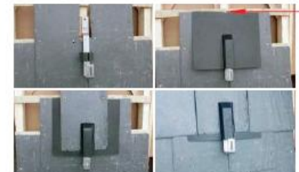
Step 4: Cut slates around the hood of the SolarFlash as per Page 4.
