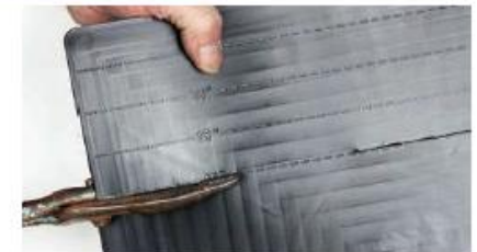
Step 2: As a guide, slate sizes are marked on the SolarFlash.
