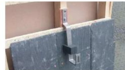
Step 1: Fix foam to bracket drop.
