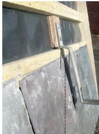
Slate roof showing 30mm clearance
